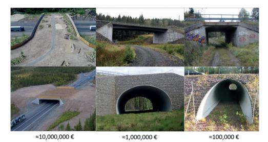
**Figure 1.** Examples of differently sized crossing structures in Sweden used by large wildlife, with rough estimates of investment costs. The precise costs depend on a number of site-specific factors, and values given are intended to serve as indications. Images by courtesy of Trafikverket and PEAB.
