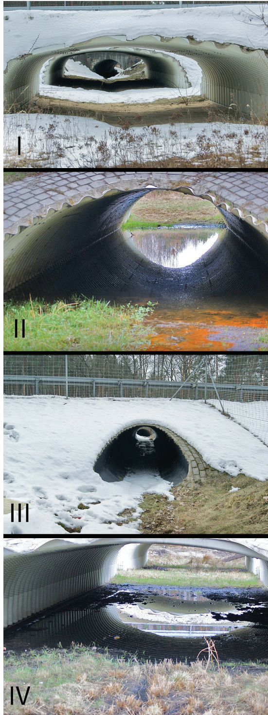
Figure 2. Monitored S3 expressway underpasses in western Poland.
