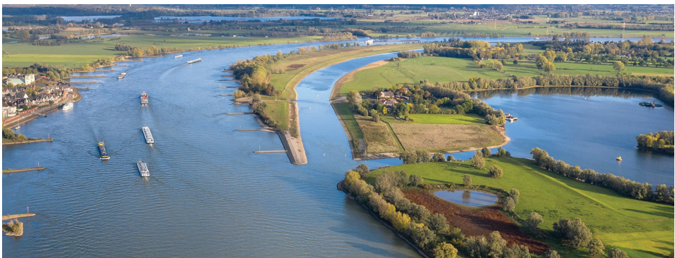
Figure 5. Rees flood spillway (Source: BAW).
