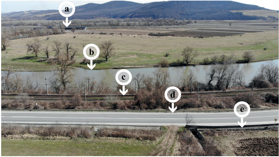
Figure 3. Cumulative impact of a highway sector between Turda and Aiud in Romania b Mureș River c railway d European road E81 and e electric fence used to keep wildlife away from the agricultural field, on the permeability of the landscape, not assessed.
