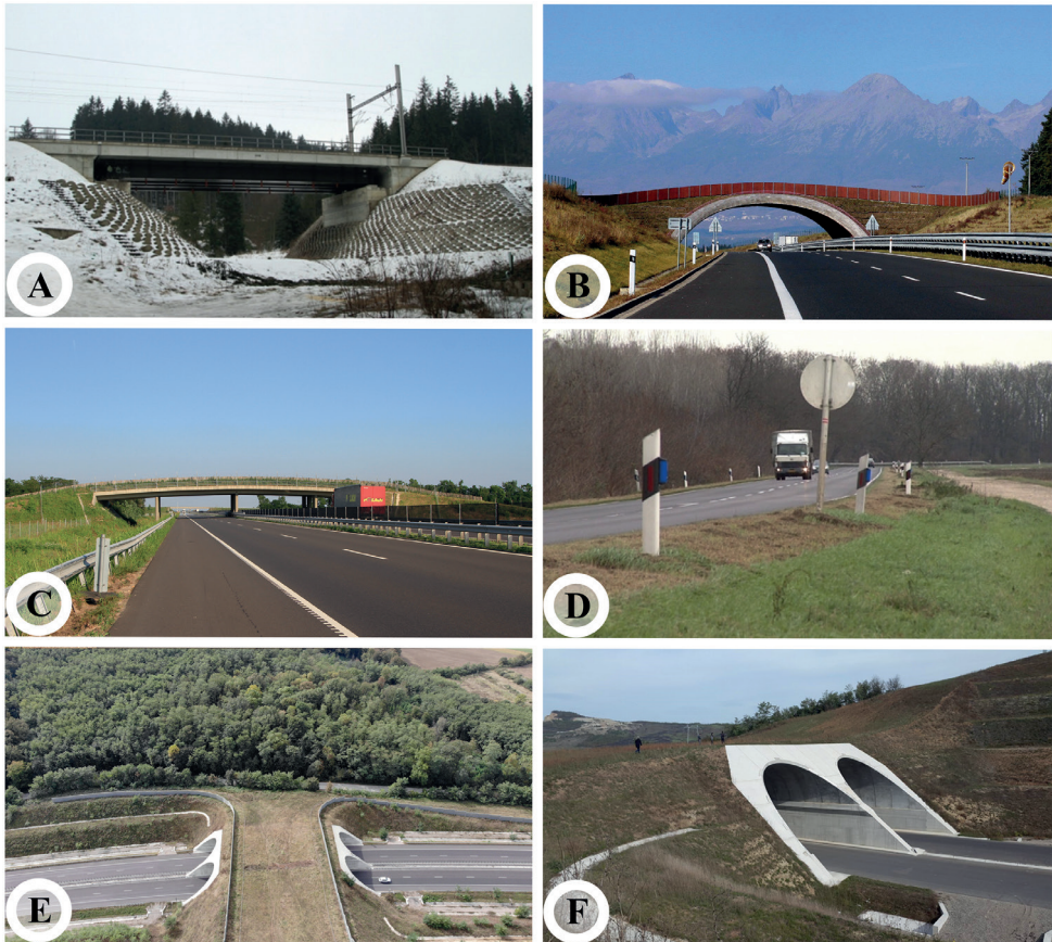
Figure 5. Positive examples of transport infrastructure development in the Carpathian countries A underpass constructed on the railway in the cadastre of the Mosty u Jablunkova close to national border in Czech Republic B overpass connecting the High and Low Tatra Mountains in Slovakia C overpass on M43 between Szeged and Nagylak in Hungary D blue retro reflectors installed on odometers on Main Road1 in Hungary E, F the first green bridge ever built in Romania on Lugoj-Deva highway, close to Brănișca Village
