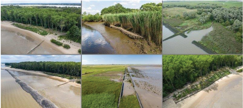
Figure 4. Biotechnical approaches to bank protection at German North Sea estuaries (Source: BAW).
