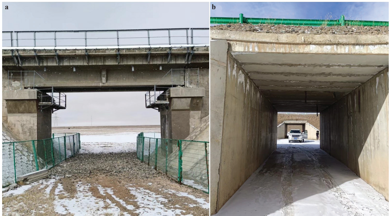
Figure 2. Photos of the underpasses a Qinghai-Tibet railway b Gonghe-Yushu expressway.
