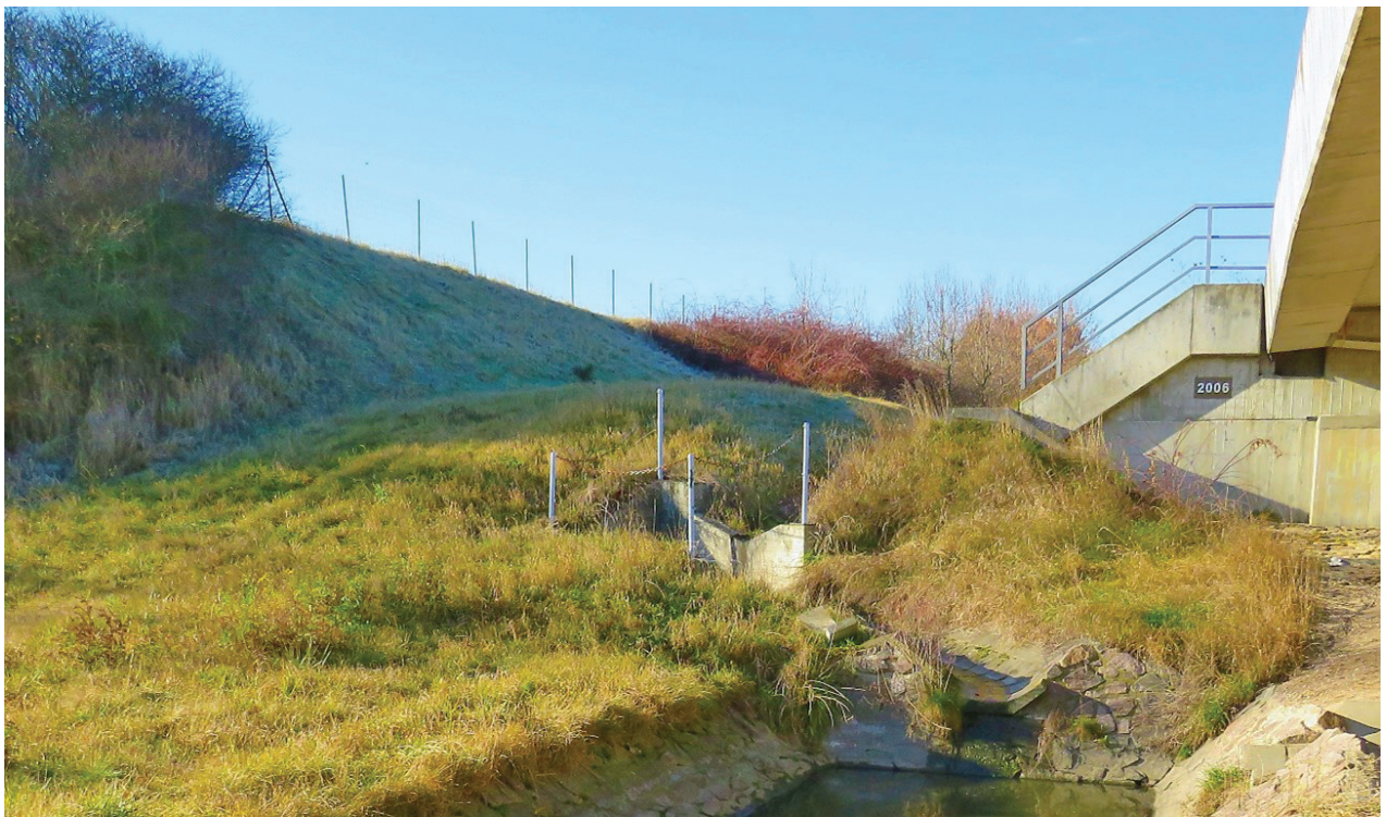
Figure A2. Inappropriate gap between the end of fencing and migration object nr. D11-066.
